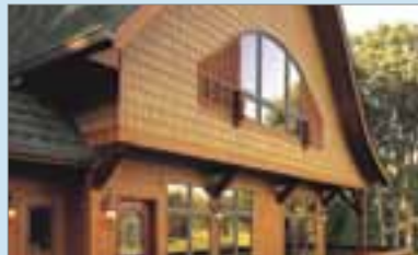
Fiber Cement Siding
